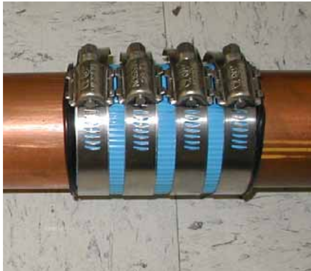
Figure 5-5. Photograph of insulating Joint using a 2" DWV coupling. A coupling with metal shield and 4 clamps is required. Some RF room suppliers will provide a special insulating coupling for use outside of room. This item is supplied by your general contractor.
